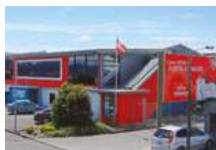
Fujitsu General New Zealand Ltd. (Nowa Zelandia)
