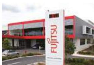
Fujitsu General (Aust.) Pty Ltd. (Australia)
