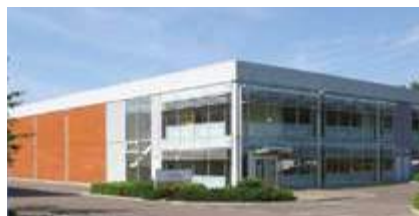
Fujitsu General Air Conditioning (UK) Limited (Wielka Brytania)
